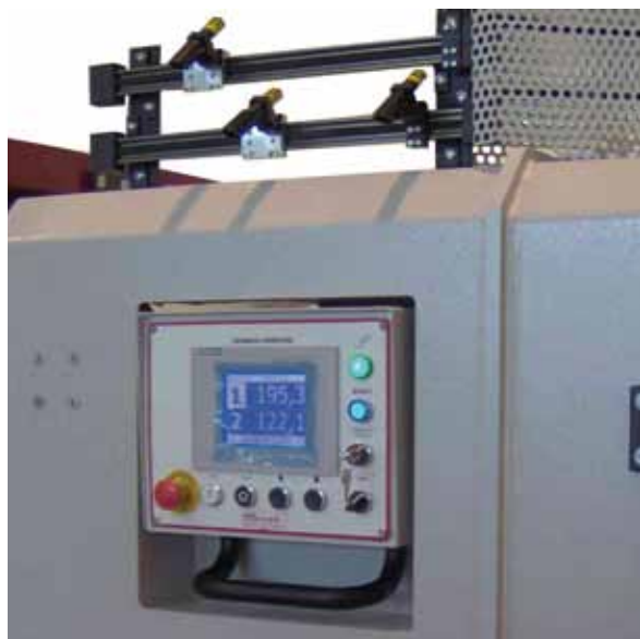
Adjustment of Inspection camera with DryLin® ZLW
